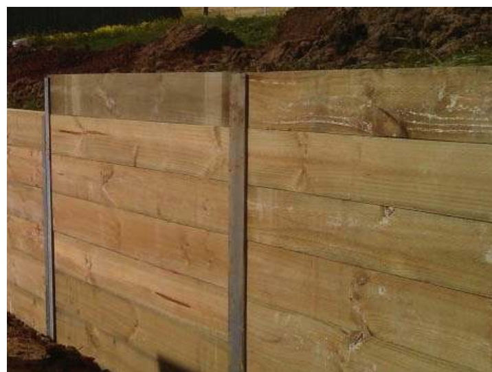
Timber sleeper retaining wall.
