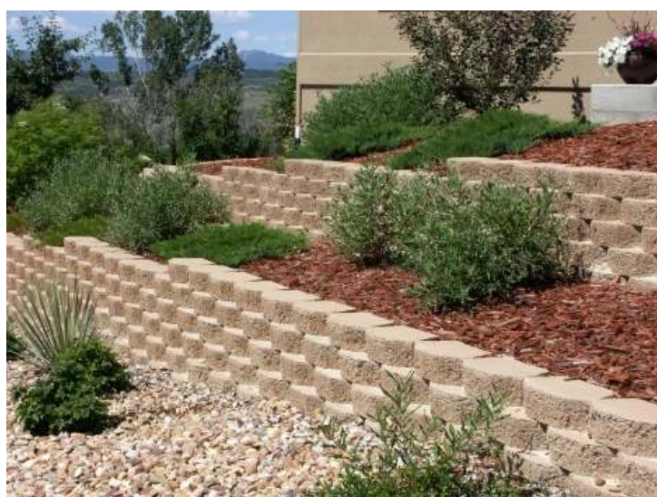
Keystone concrete block retaining wall.
