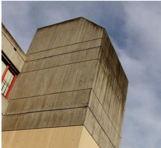
Figure 4. Detail showing off form concrete construction at scale. Source: Diahne Sullivan, 2012.
