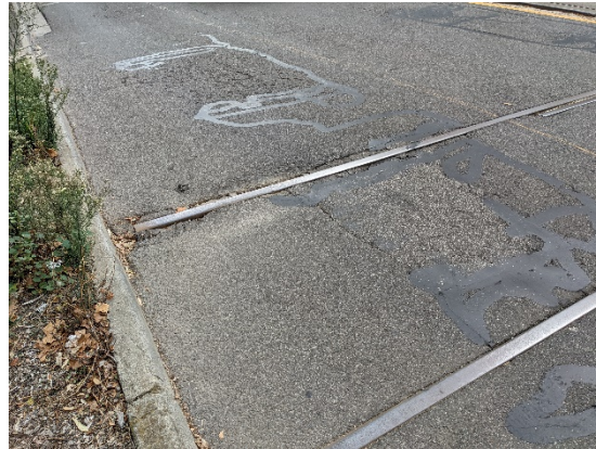
Figure 68 Detail of pavement failures at Lygon Street
