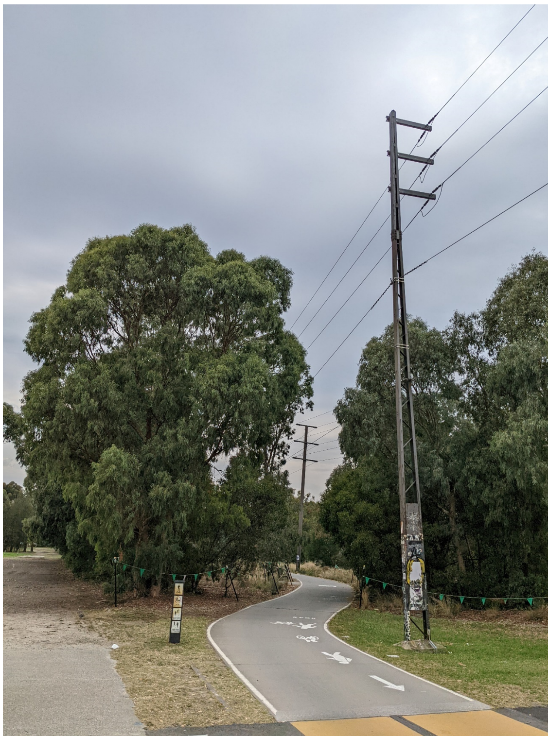
Figure 77 Historical power stanchion in Janet Millman Reserve; many of these steel truss stanchions were formerly piers in the overhead traction power supporting structures of the electrified railway. The anti-climb plates near the base are a natural fit for identity signage, interpretation or artwork, and could be presented in sequence across the more than twenty accessible stanchions in the parklands
