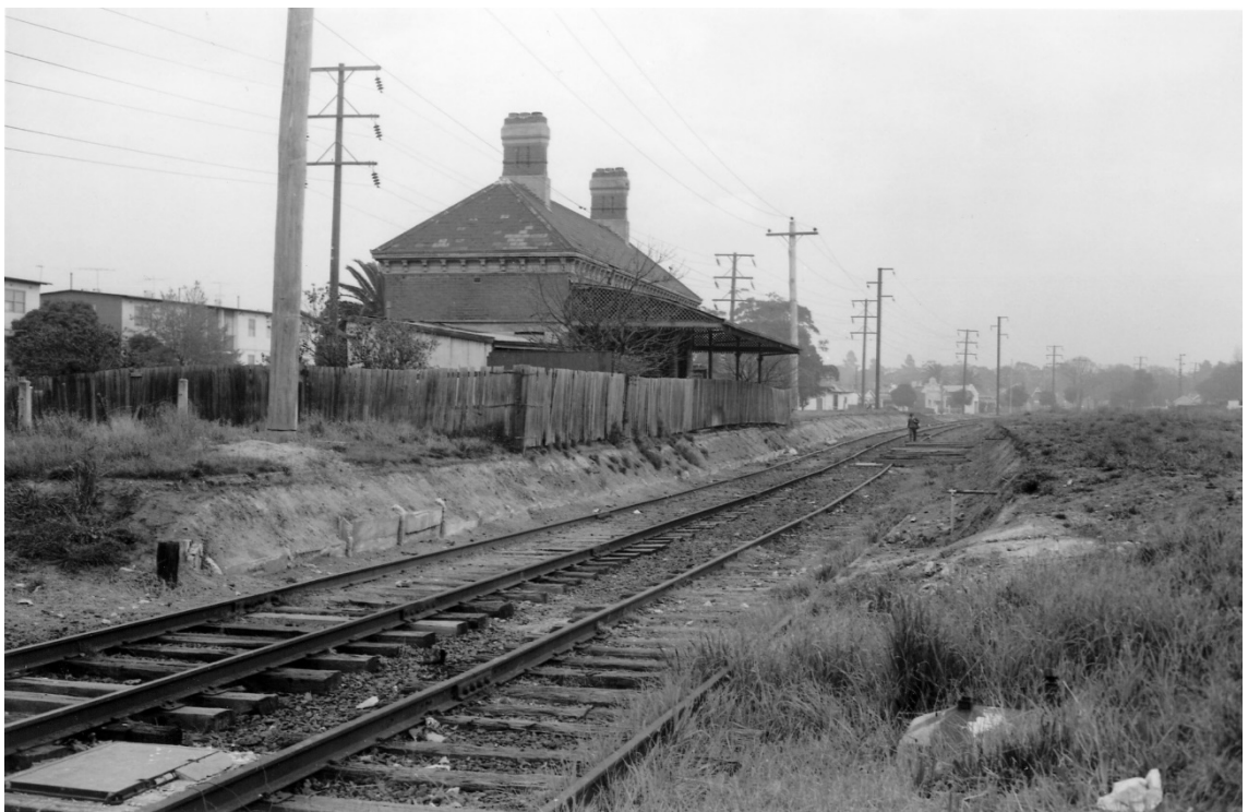
Figure 27 North Carlton Station building, fenced off and reused as railway worker housing, c. 1960s; note the disused north track and removal of overhead electrical equipment and supports Source: Public Records Office Victoria
