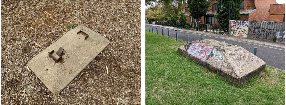
Figure 78 Two examples of small and large-scale concrete footings which remain in the parklands; at left a small footing for a power stanchion, at right a very large concrete footing whose original purpose is not known
