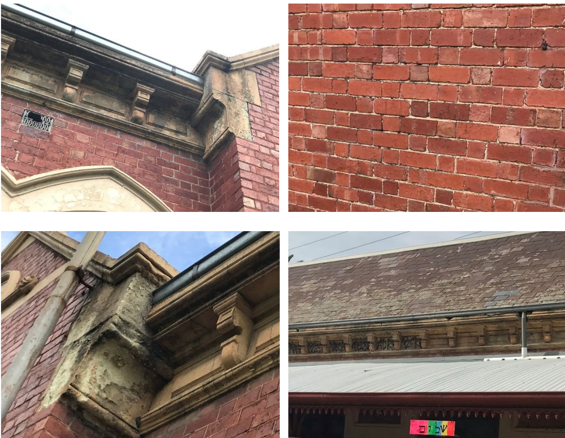
Figure 64 Detail photos showing current condition of rendered cornice, stone brackets, weathered masonry, roof slates and improper rainwater goods
