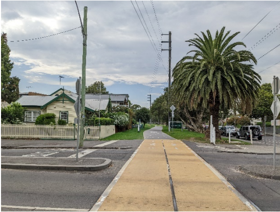
Figure 65 Bowen Cres trail priority crossing with embedded track
