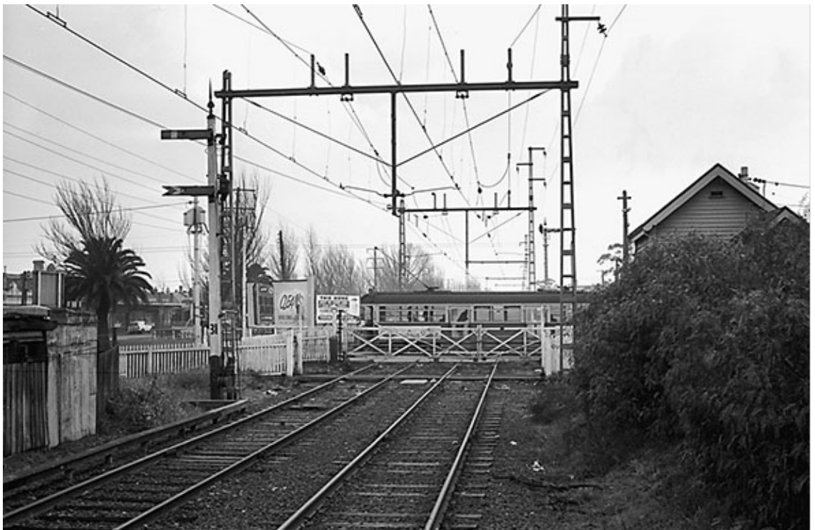
Figure 23 Overhead support structures and electrical stanchions at a major road crossing, 1963 Source: Courtesy John Thompson
