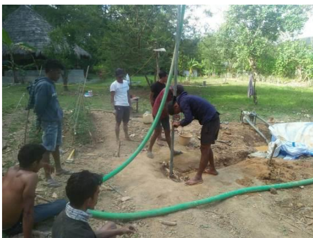
Installing water bore at Kadalak Dame Garden
