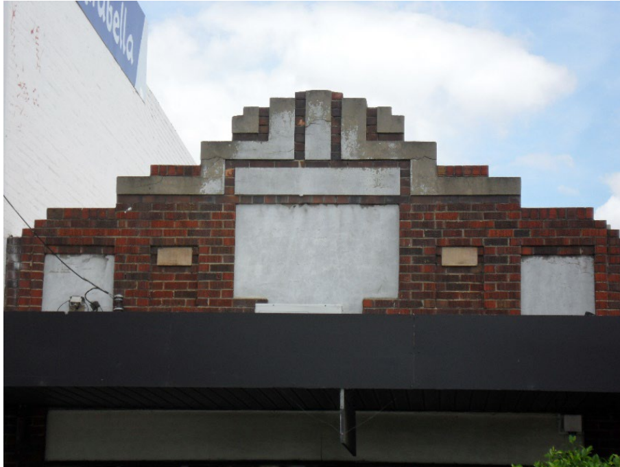
Figure 2. Detail of parapet, showing distinctive stepped profile and geometric patterning. (Source: GML Heritage Victoria t/as Context 2017)
