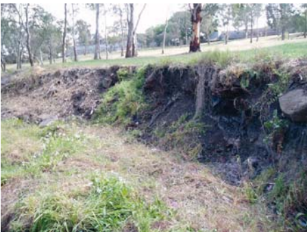
Photo 2: Eroding fill embankment upstream West Street Drain (2007)
