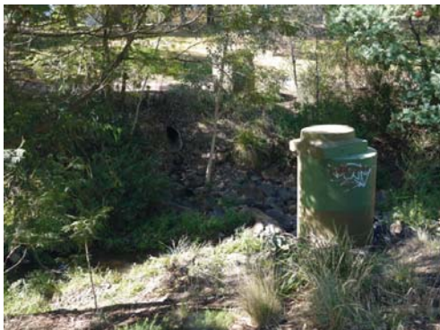
Photo 15: Exposed sewer pit Gavin Park North
