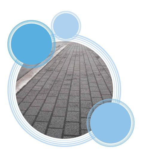
Permeable pavements allow stormwater runoff to infiltrate to underlying soils rather than running off hard surfaces and into the stormwater drainage system. Permeable pavements are used for a wide range of purposes including:
