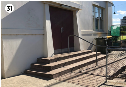
31 ISSUE: Pedestrian access into and around buildings is non compliant with current building codes. OPPORTUNITY: Provide compliant pedestrian access with upgraded or new building entrances and linked walkways.
