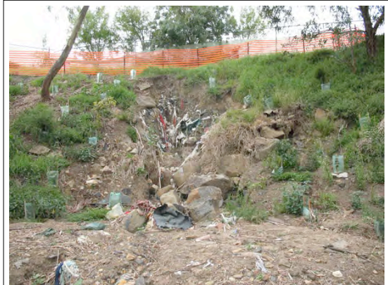
Photo 7 Overland flow erosion - Coburg Hill
