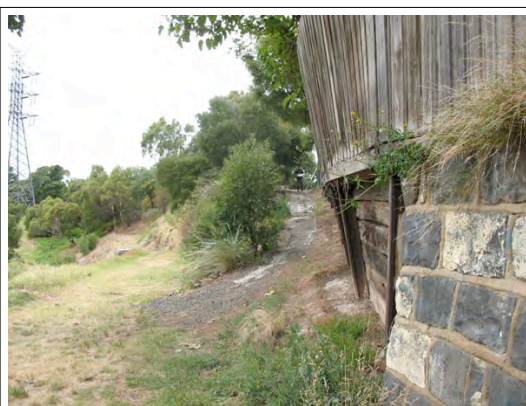
Photo 37 Failing private property retaining wall at Jenkins St
