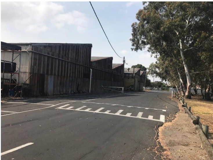
Figure 3: Western boundary of 16-20 Sheppard Street
