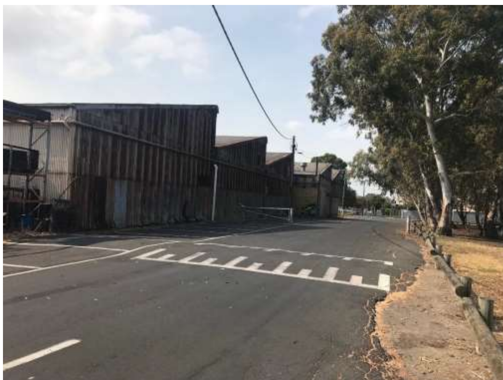
Figure 3: Western boundary of 16-20 Sheppard Street
