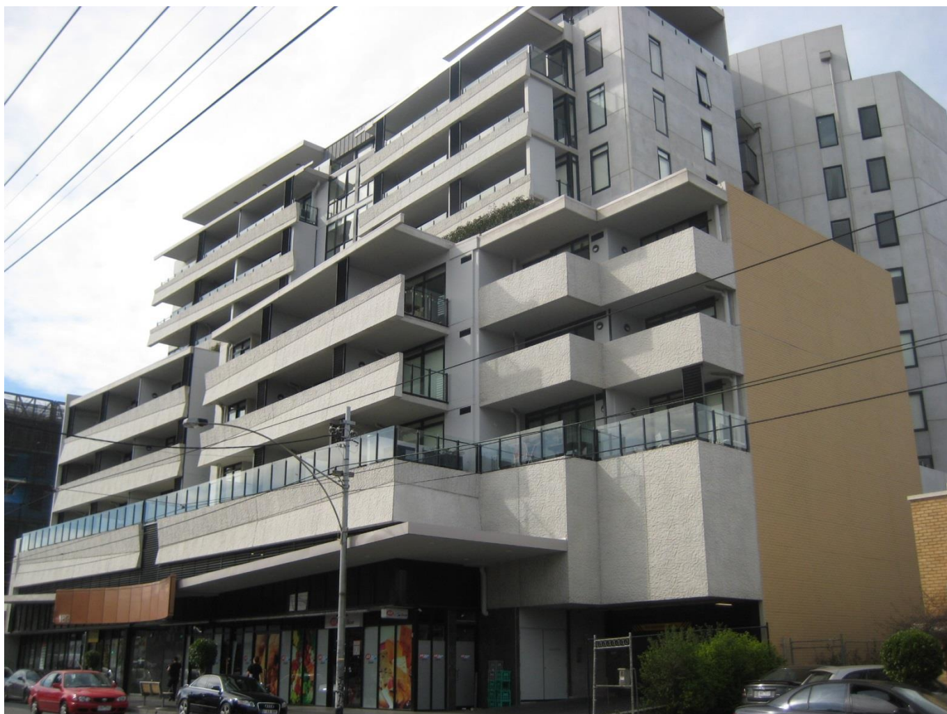
'Elvera' 330-340 Lygon Street, Brunswick—modest additional setback combined with uniform architectural expression fails to create distinctive or recessive upper form
