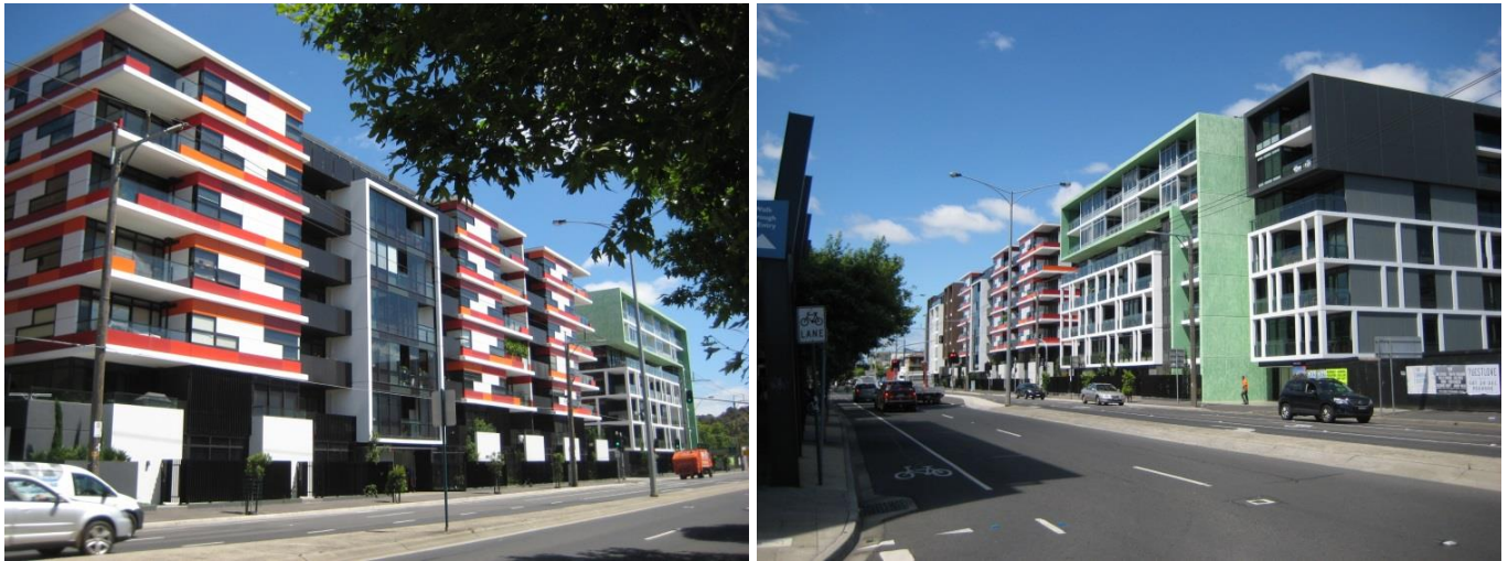
Buildings in Burnley Street, Richmond, whose height is equal to the road reserve width.
