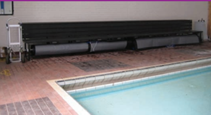
POOL BLANKETS IN USE AT FAWKNER LEISURE, AND STORED UNDER BENCH SEATING. STAFF TRAINING HAS BEEN A KEY TO ENSURE THE POOL BLANKETS ARE USED APPROPRIATELY.
